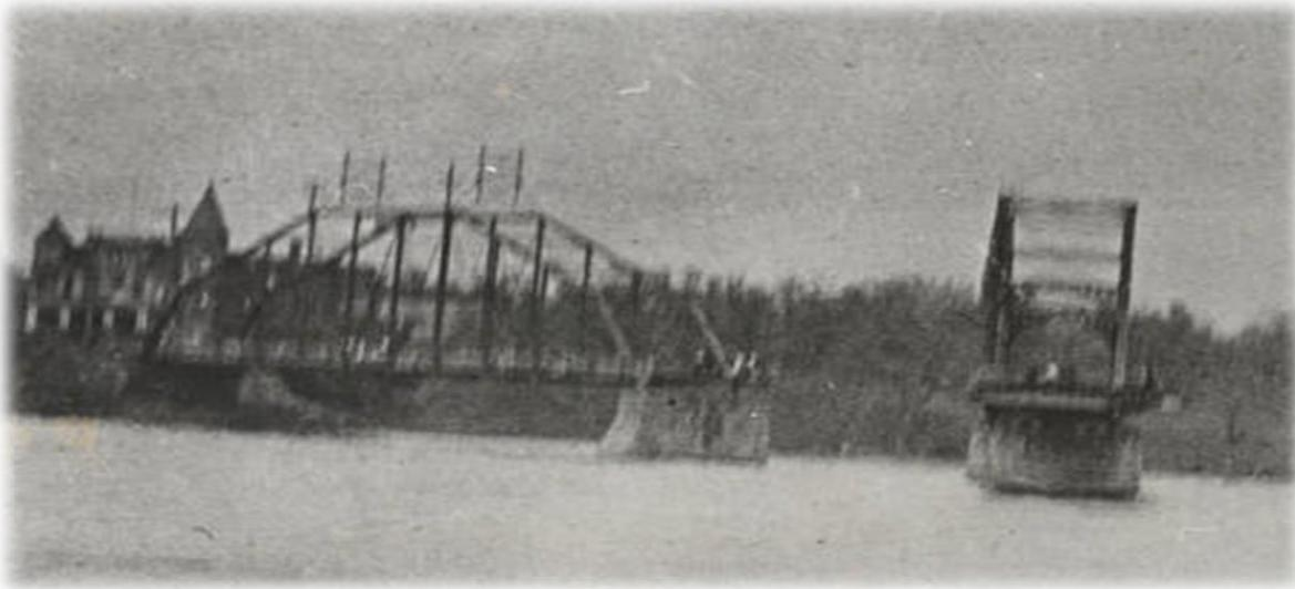
The first bridge to span the Mississippi River between Champlin and Anoka opened in 1884. It was a spring bridge with the center section turning on a central pier, like a hinge on a door, to allow boat traffic to pass alongside the open bridge. It was 900 feet long with an 18 foot wide roadway and was constructed of iron with a wood deck and rested on Kasota stone and granite piers.
