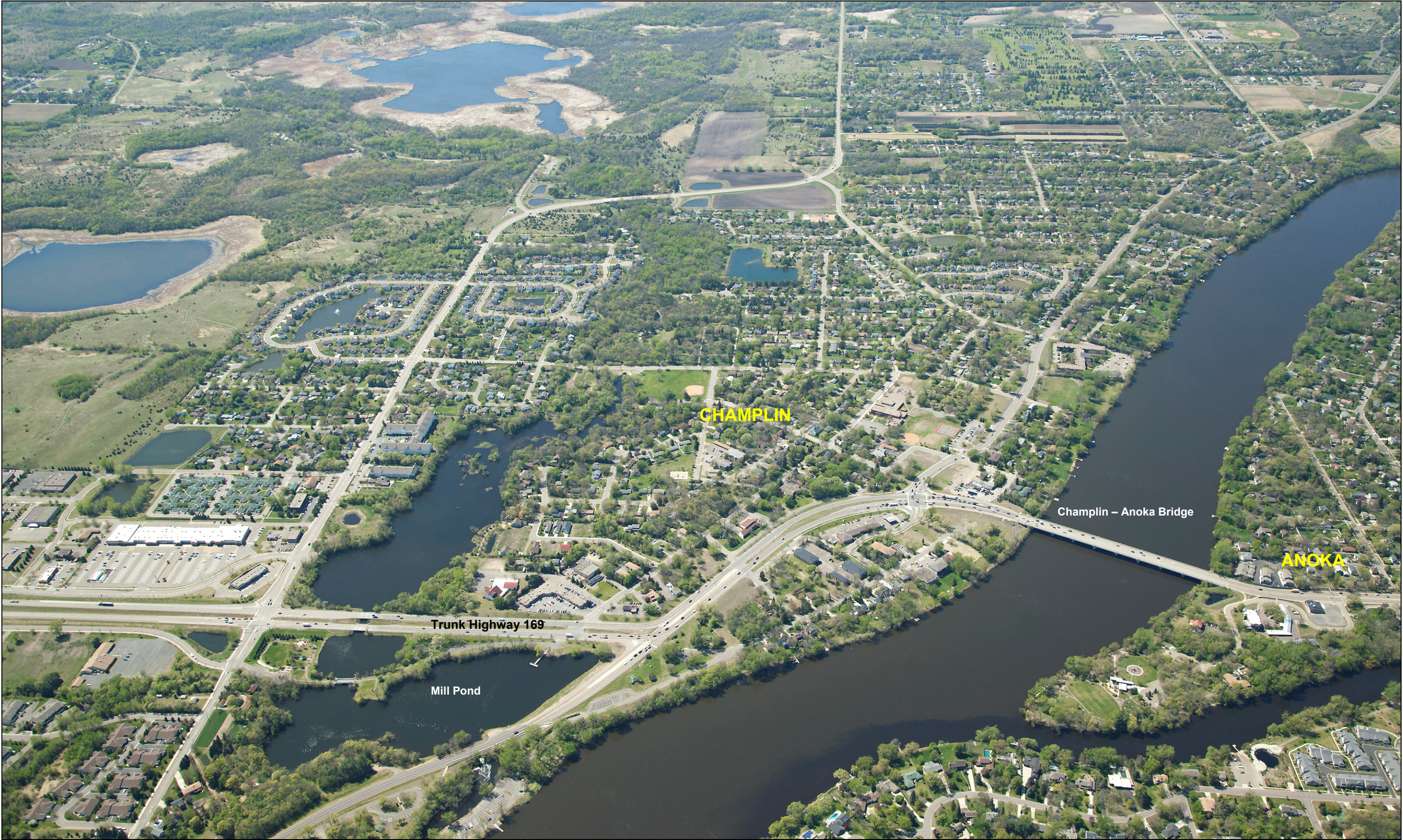
Mississippi Crossings Aerial - 2012
