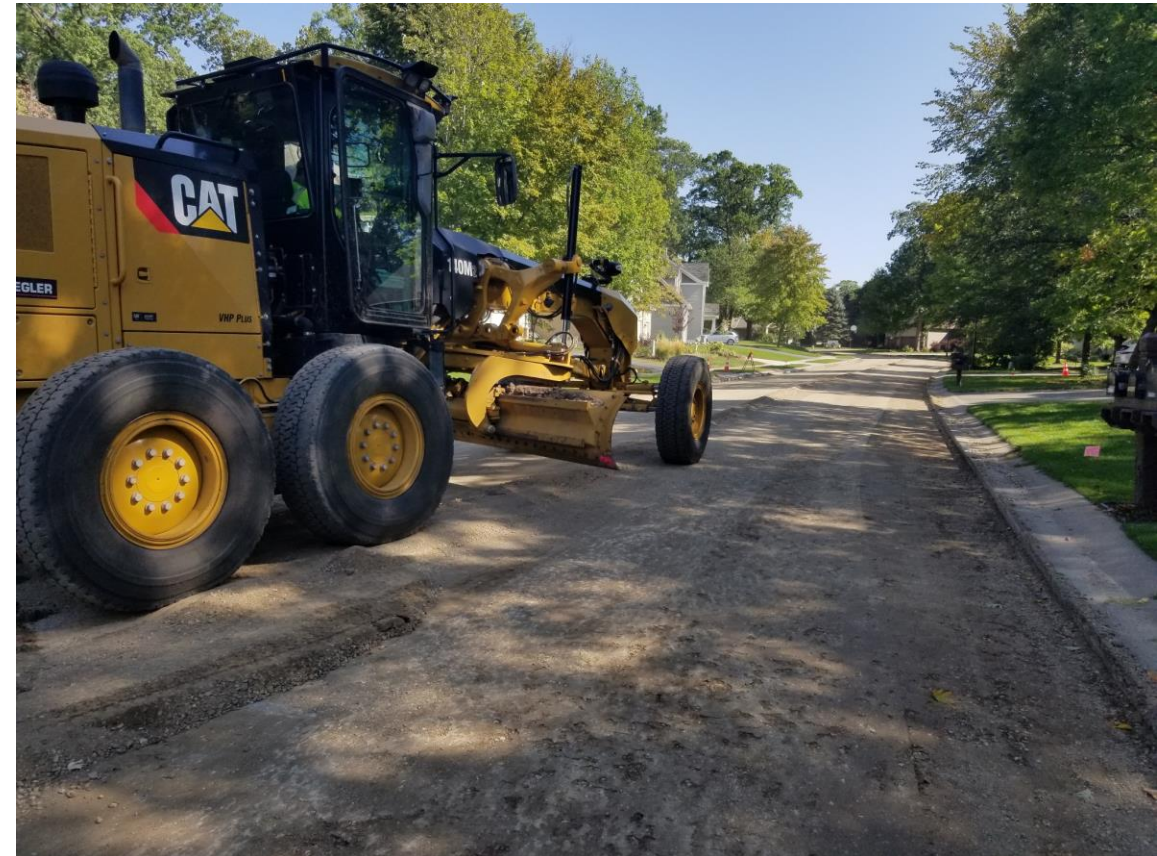
Pavement Removal and Grading
