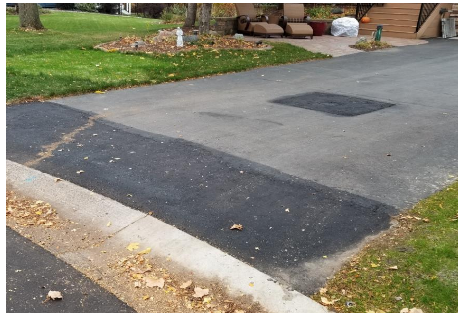
Spot Curb Replacement and Curb-Stop Repair Areas
